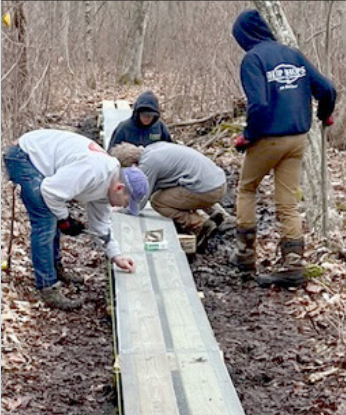
Work at a particularly mucky stretch of the Yellow Trail culminated in a boardwalk to improve the hiking experience at the Boggy Hole Preserve.
