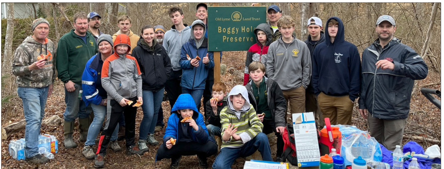
The hardworking crew rests after a gratifying morning of installing a bridge and two walkways. Leader Brenden Landry is second from the right.
